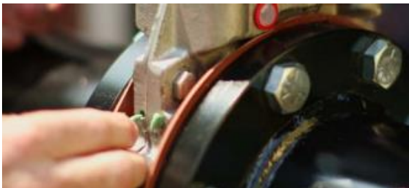
Step 2b: Insert one packing pellet (approx. 1" length) in the other hole.
